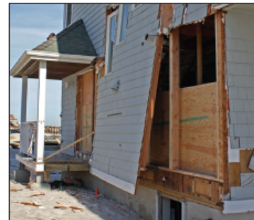
Figure 1: Back wall failure due to flood level above the lowest floor of a house in Ortle Beach, NJ
